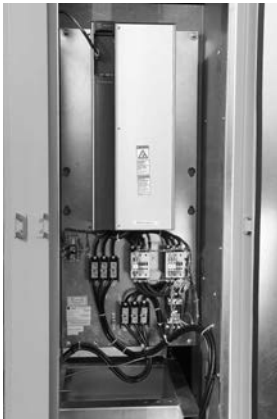
Figure 7. Variable frequency drive
