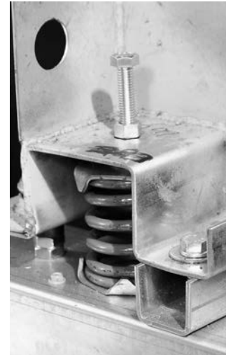
Figure 6. Spring isolation
