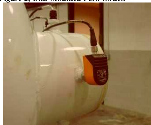
Figure 2, Unit-Mounted Flow Switch
