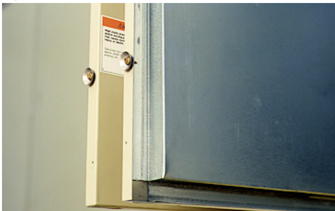
Figure 1: Full Double-Wall Construction
