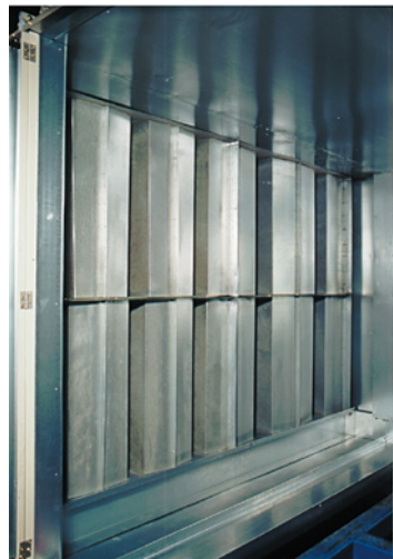
Figure 18: Factory-Installed Sound Attenuators
