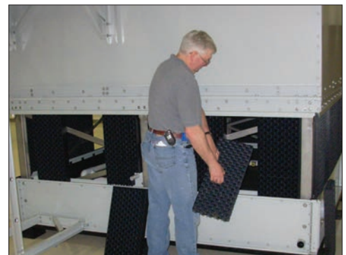
Combined Inlet Shields
