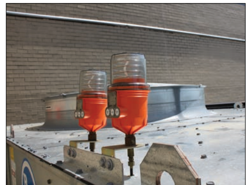
Automatic Bearing Greasers
