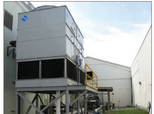
EVERTOUGH™ Construction Installation
