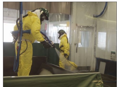
Application of TriArmor® Corrosion Protection System
