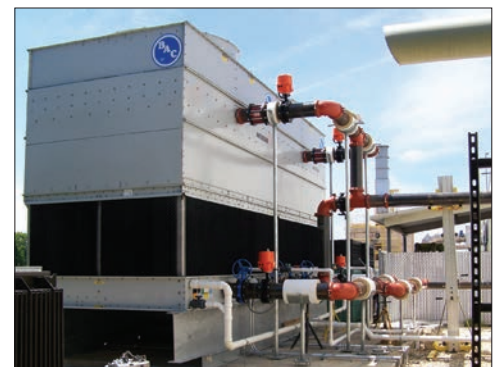
Side Inlet Connection
