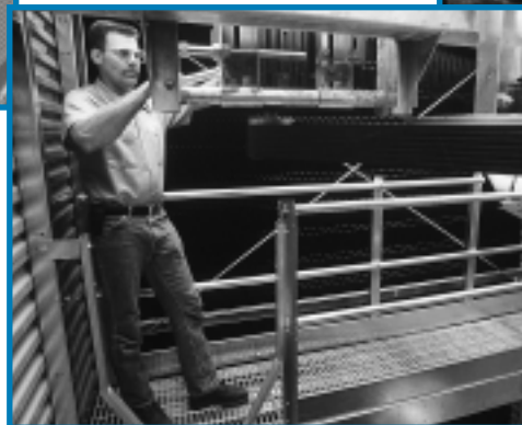
Internal ladder and service platform
