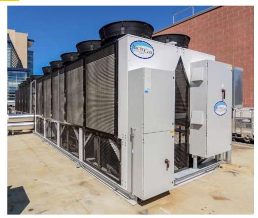
Chiller Base Model: ACA220BT3512F-FC-460V Air Cooled Chiller, 230 ton
