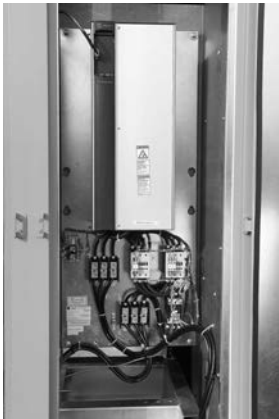
Figure 7. Variable frequency drive
