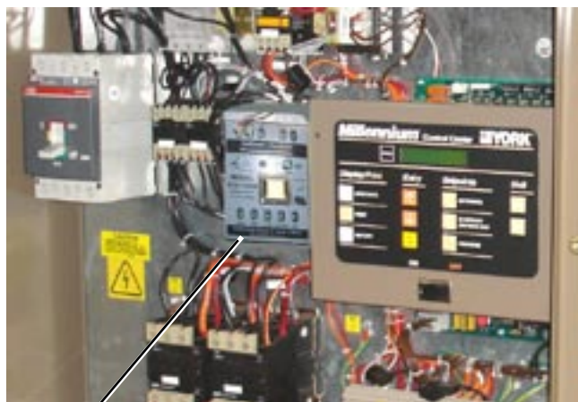
FIG. 18 – TYPICAL VFD LOCATION
